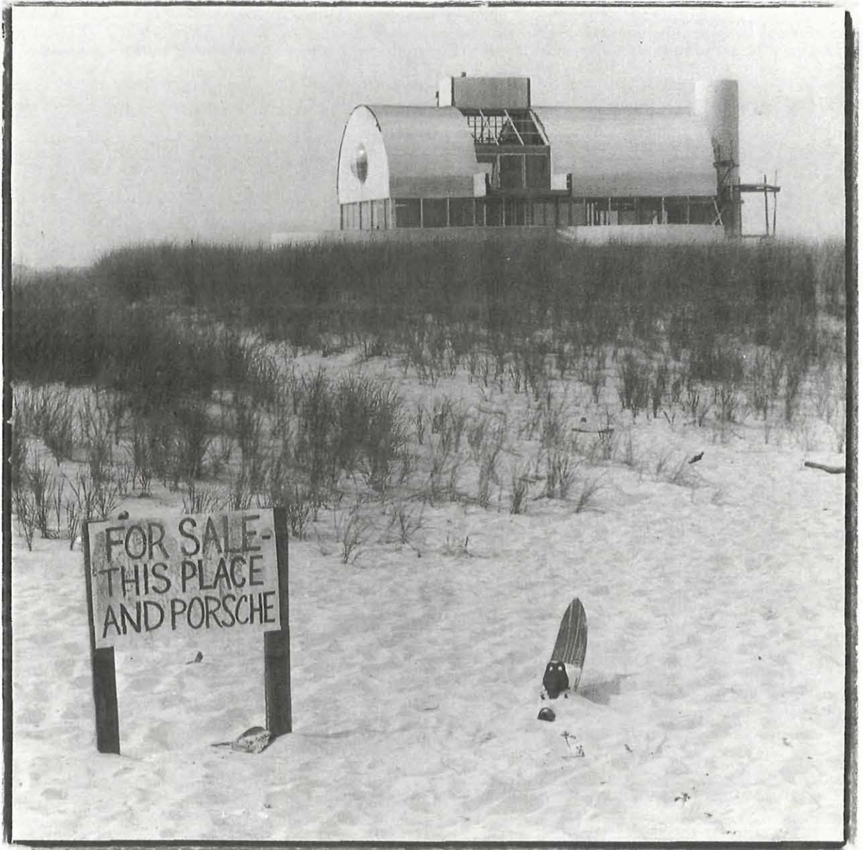
A half-finished beach house is abandoned, inundated with sand. “The contractor disappeared with my money, and the banks raised the interest on my loan. I couldn’t keep up, so I said, ‘The hell with it.’” —An advertising creative director, Southampton, Long Island
